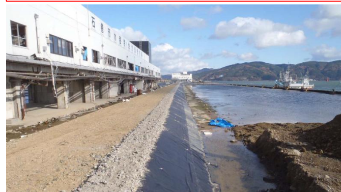
The level raising of the area of fishing ports facilities to stop flooding hinterland
