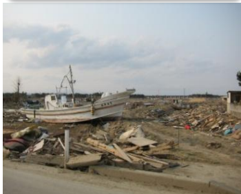
Damaged fishery processing facility
